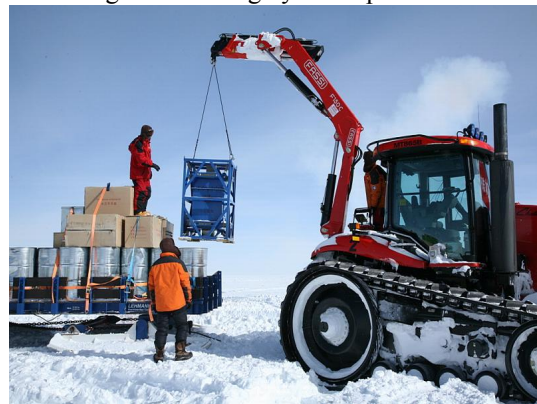
Figure 12 lifting by CAT
