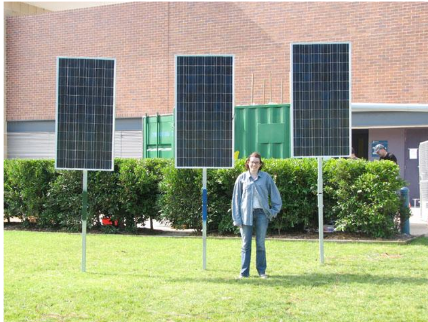
Fig. 3. One of the two solar arrays erected at UNSW for testing.
